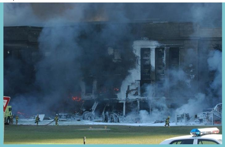
The exterior columns on the left of the damaged exterior section - below - are shattered, with the dangling rebar bent outward.
