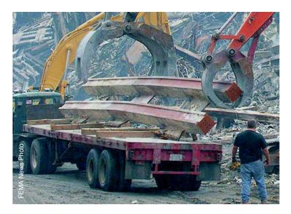
**Figure 3-10** Two columns still attached to the three plates that made a pre-fab unit.
