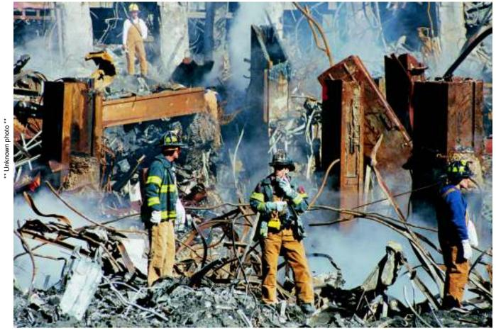
Figure 3-5 The core column in the center appears cut by a torch. The workers cut the steel so quickly that it is difficult to determine which damage was from them.
