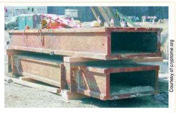
Figure 3-6 Core columns, sliced and ready to sell as scrap. This photo was taken at the WTC on October 3rd, 2001.
